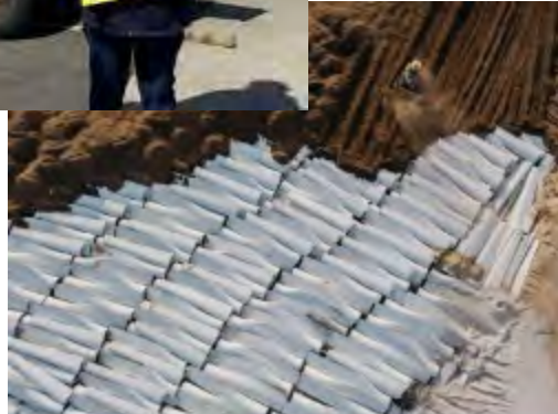
Fragments of wind turbine blades await burial at the Casper Regional Landfill in Wyoming. Photographer: Benjamin Rasmussen for Bloomberg Green
