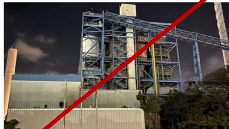
Retirement of the 180-megawatt AES Hawaii coal plant on Oahu ends the use of coal for power generation in the state. Closure of the plant — one of the largest emitters of greenhouse gases — aligns with Hawaiian Electric's overall plans to decarbonize its energy systems. Photo courtesy of AES.
