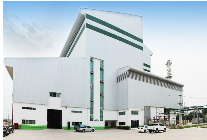
6MW of RDF Power Plant
