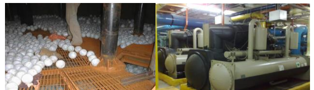
District Cooling with Thermal Storage
