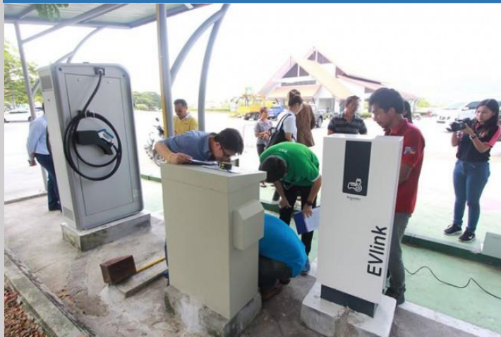
Install EV charging station
