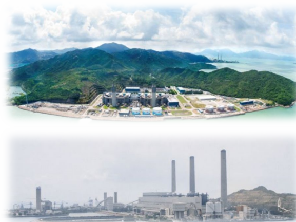
(1 x 550 MW and 1 x 380MW )
